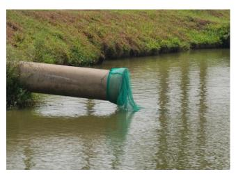
Figure 3: Protection of inlet pipe with a mosquito net bag
